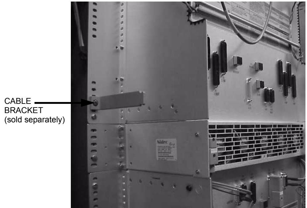
Figure 1-6 Cable brackets
