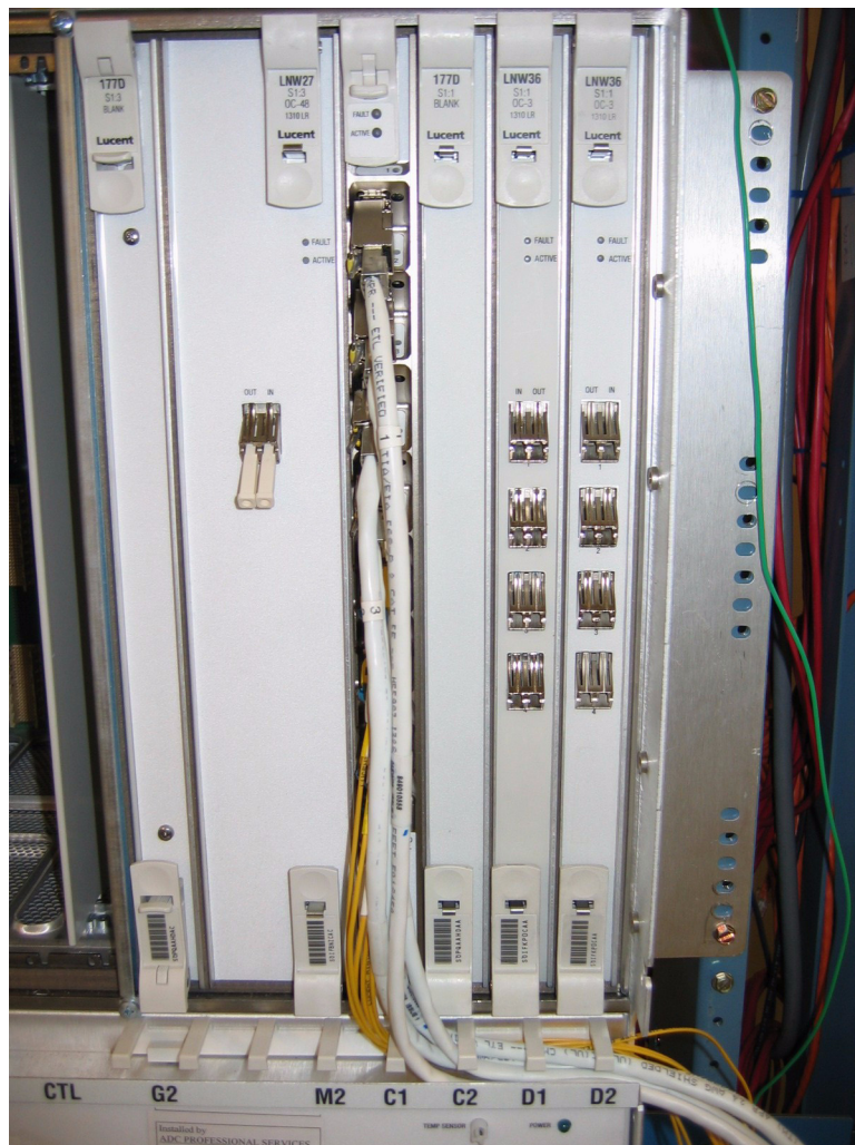
Figure 1-19 Ethernet cable routing to faceplate SFP modules
